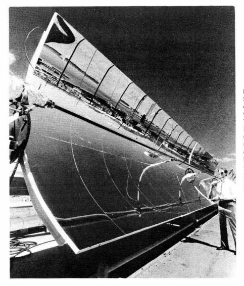
IMPROVED EFFICIENCY — Sam Martin (2323), project engineer, stands beside the Engineering Prototype Trough, a new solar collector that has shown a solar-to-thermal conversion efficiency of 60 percent, some 10 to 20 percent higher than earlier collectors. The prototype is designed to be readily mass produced. See article on Page Four.
